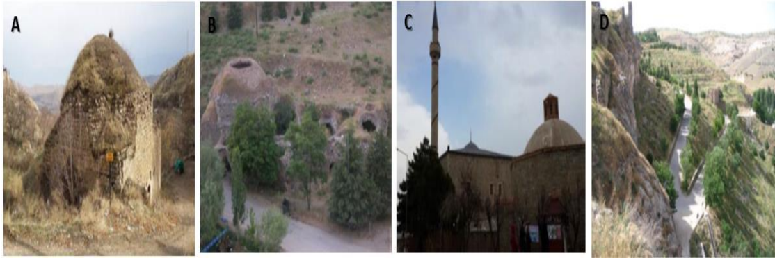
Fig. 7. Harput's baths (A: Hoca bath; B: Kale bath; C: Cemşit bath; D: Dabakhane bath)
