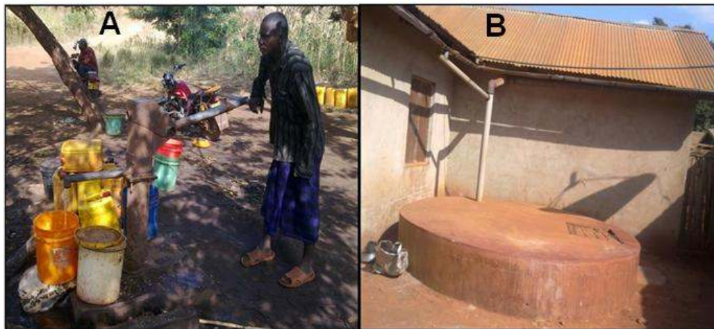
Plate 1. Bore hole (A) and rain water harvest (B) as sources of water in Kabuku Ndani ward
